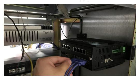
Our brackets allow for the installation of non-rack mount switches.
