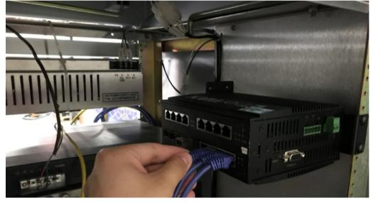
Devices can be attached directly to the bracket.
